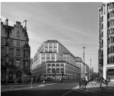
Looking west, the bulky "prow" end is more like a steamshovel plough
